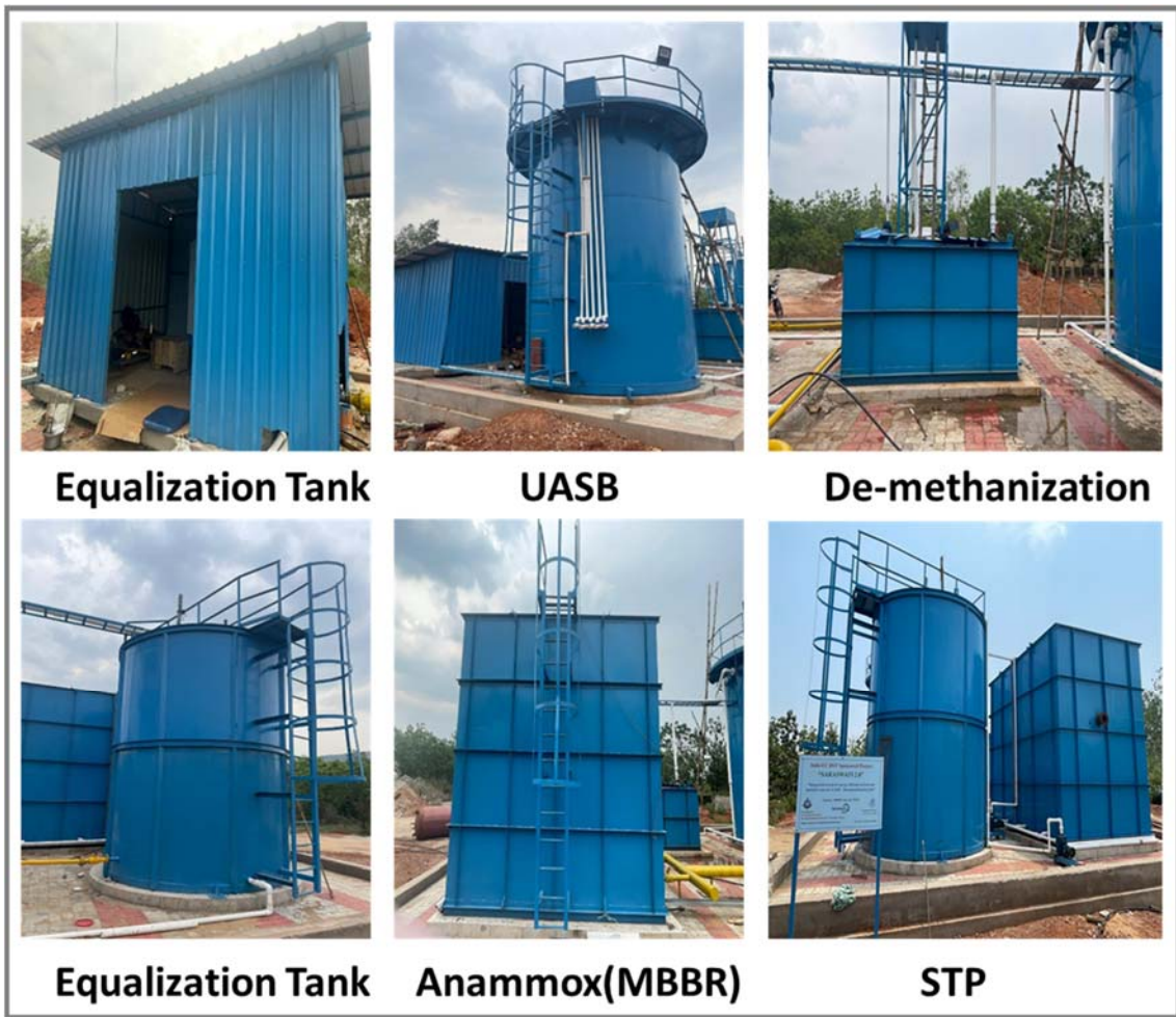
Figure 3: Construction and installation of pilot plant
