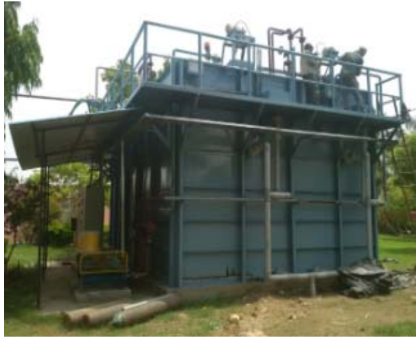
Figure 2 – Construction and installation of pilot-scale SBR
