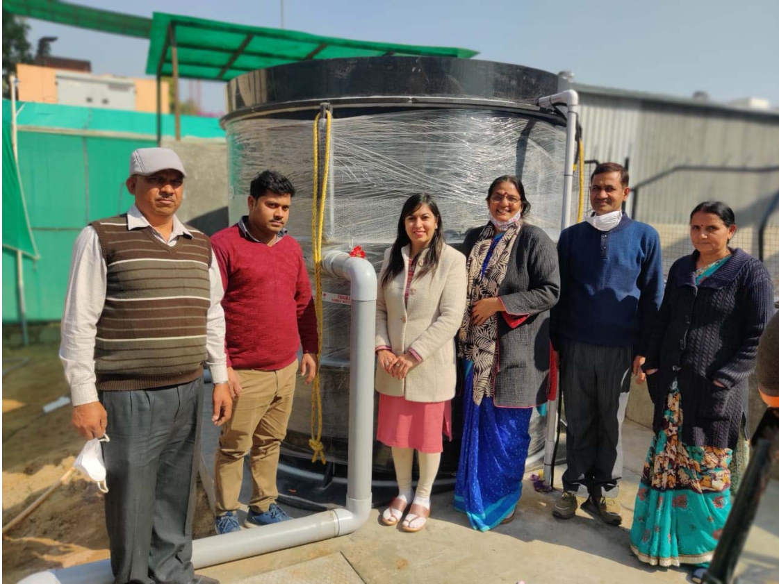
Picture above: Mars 3000 plant implemented at B.Lal
